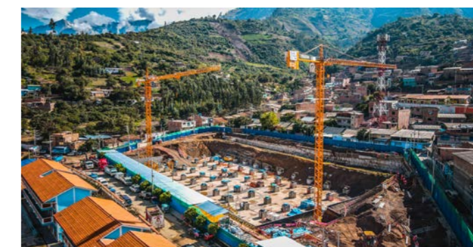
Peru Reconstruction (Hospitals)
