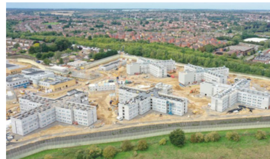
Five Wells Prison, Wellingborough
