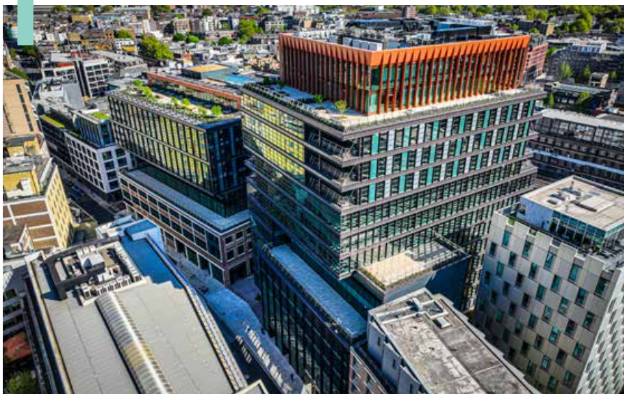
Timber Square London – UK
