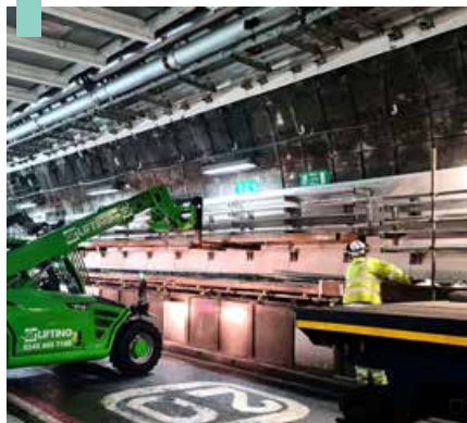
Cargo Tunnel Heathrow Airport – UK
