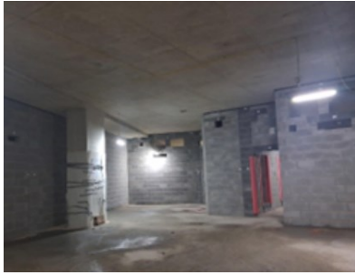
Blockwork in the basement
