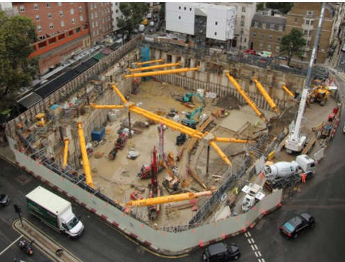
GSHP being installed on site by the red bore machines shown in the photo above
